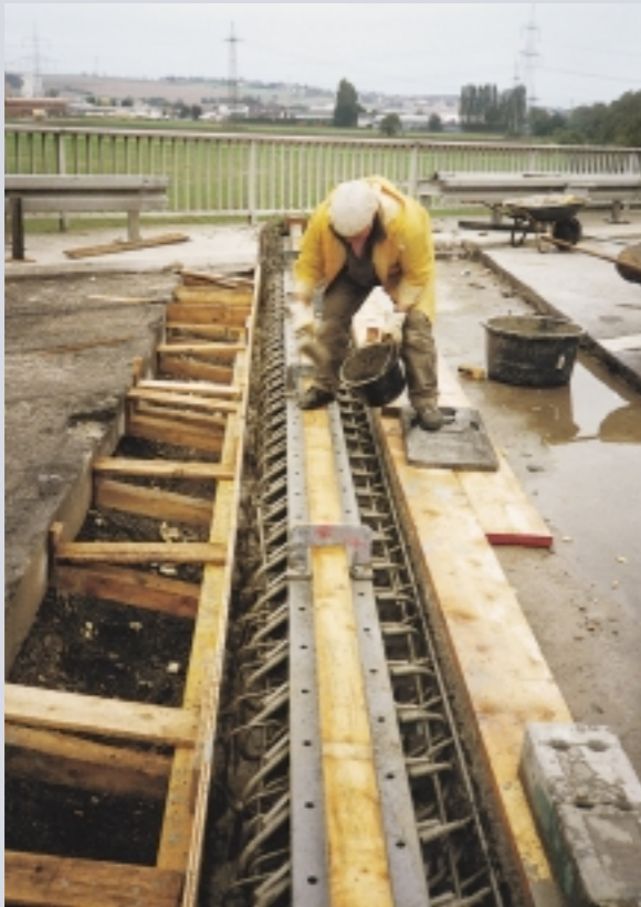
Covering of the sealing element before concreting
