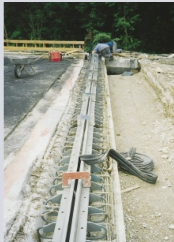
Assembly of an expansion joint construction type D80
