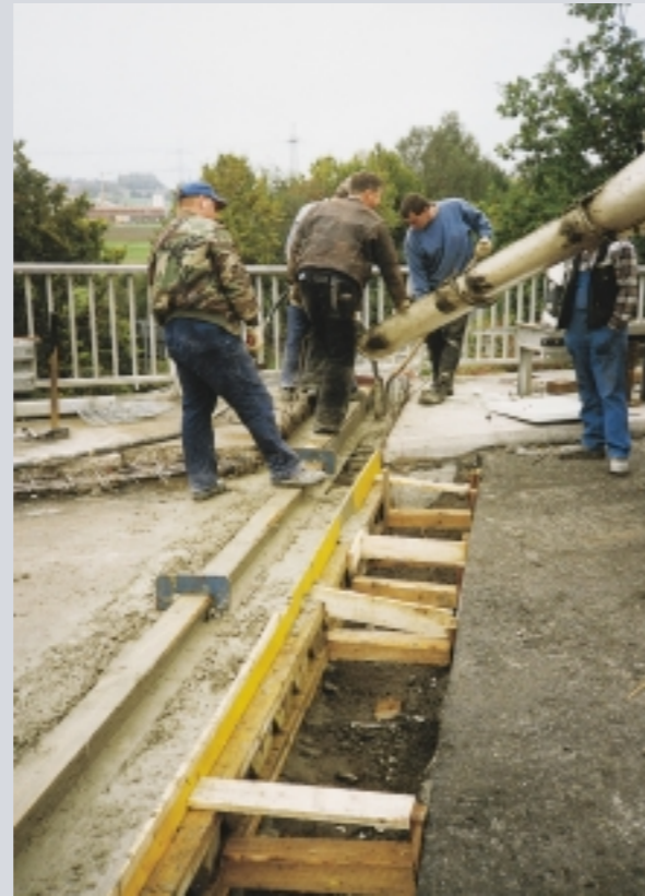
Concreting the recesses
