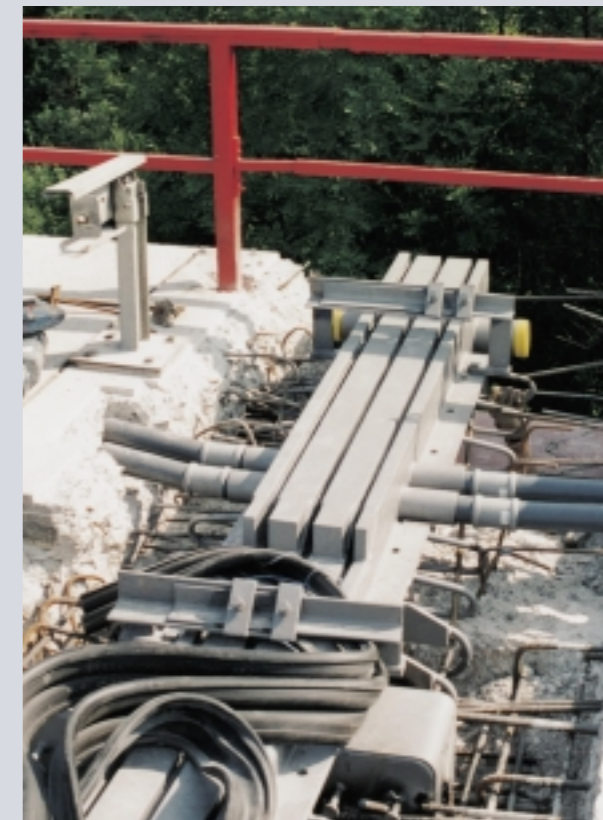
Expansion joint in the parapet cover with cable conduit
