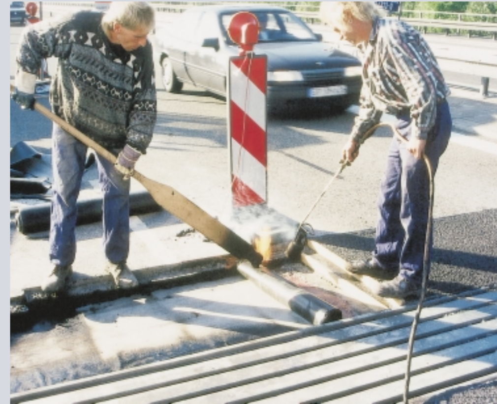
The sealing is glued on hot
