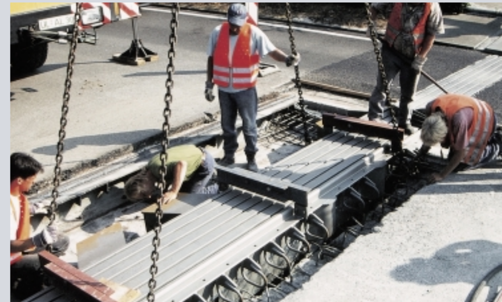
Insertion of the complete expansion joint into the construction joint
