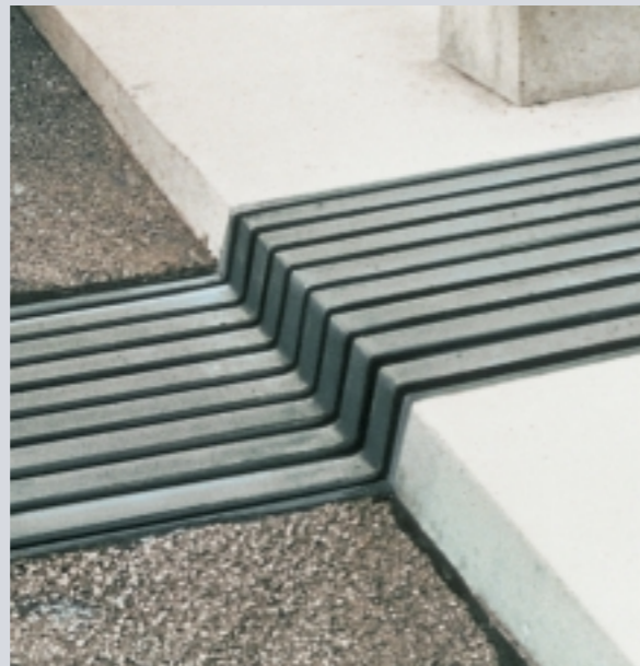
Design of the kerb unit (carriageway – footway)
